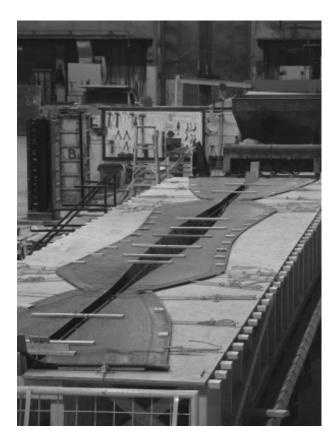
Figure 3. Installation of fabric formwork sheet.
